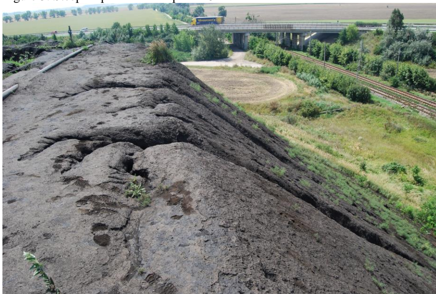
Obr. 3: Strmé svahy so sklonom 45^\circ Figure 3: Steep slopes with a slope of 45^\circ
